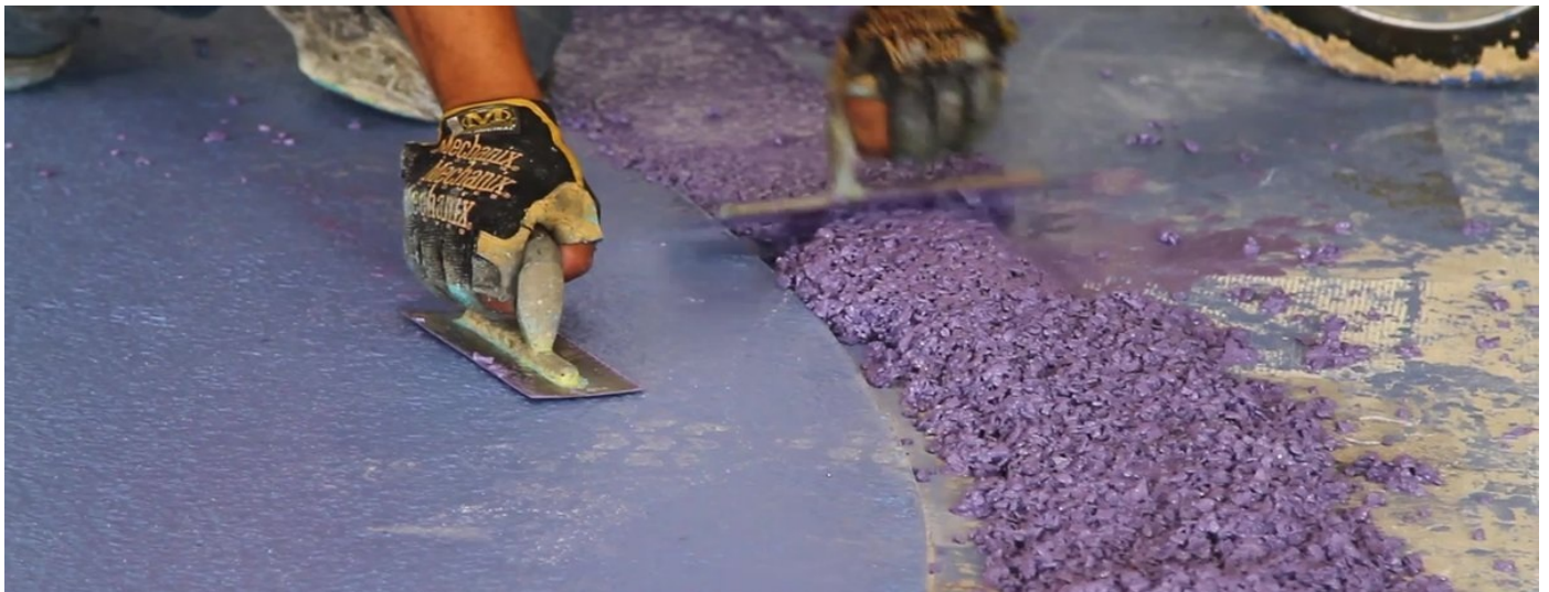
Resinous flooring applied on site — the outcome of decisions made months earlier.
