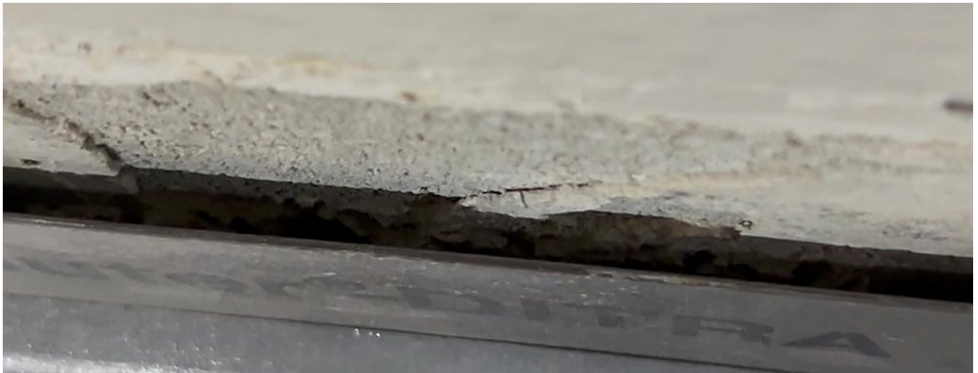
Old adhesive residue being removed ahead of a new installation.
