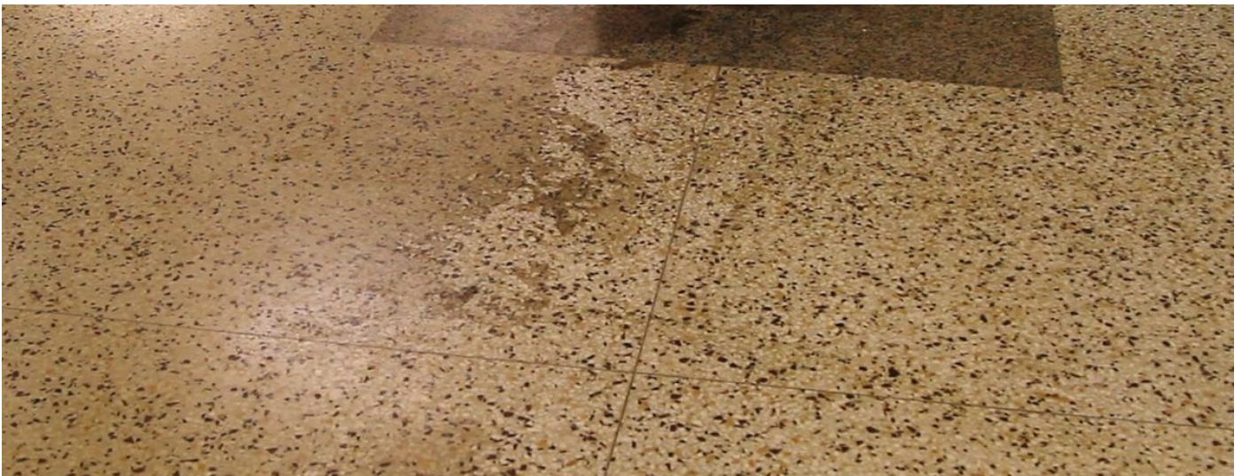
Ceramic tile in a heritage building — specified for a service life measured in decades.
